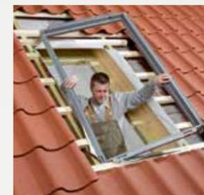
An insulation collar further reduces heat loss and eliminates cold bridges. This makes it quick and easy for you to be compliant with building regulations.
