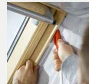
The vapour barrier helps prevent the build-up of condensation in the roof construction. Ideal for making your installation air tight.
