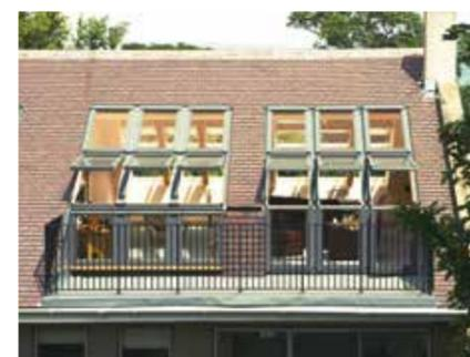
The Top-Hung upper element and side-hung lower element combine to produce a doorway to the outside terrace. All other upper elements in the combination are Top-Hung whilst the vertical elements are fixed.
