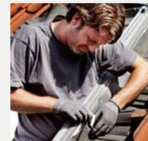
An underfelt collar ensures a weather tight seal and eliminates cold bridges. Again, this helps you to meet building regulations.
